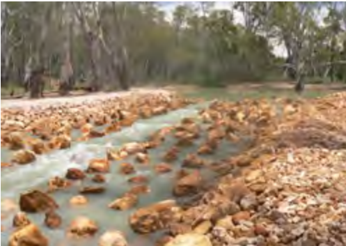
Fish-friendly rock ramp which also helps reduce erosion. Photograph: Jason Higham.
